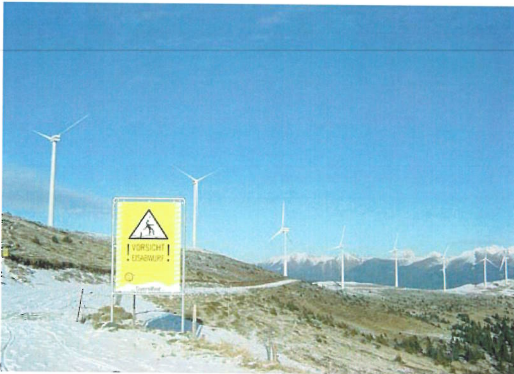
Figure 9. Warning against shedding ice fragments at Tauernwindpark in Austria. Photo from http://www.tauernwind.com .
