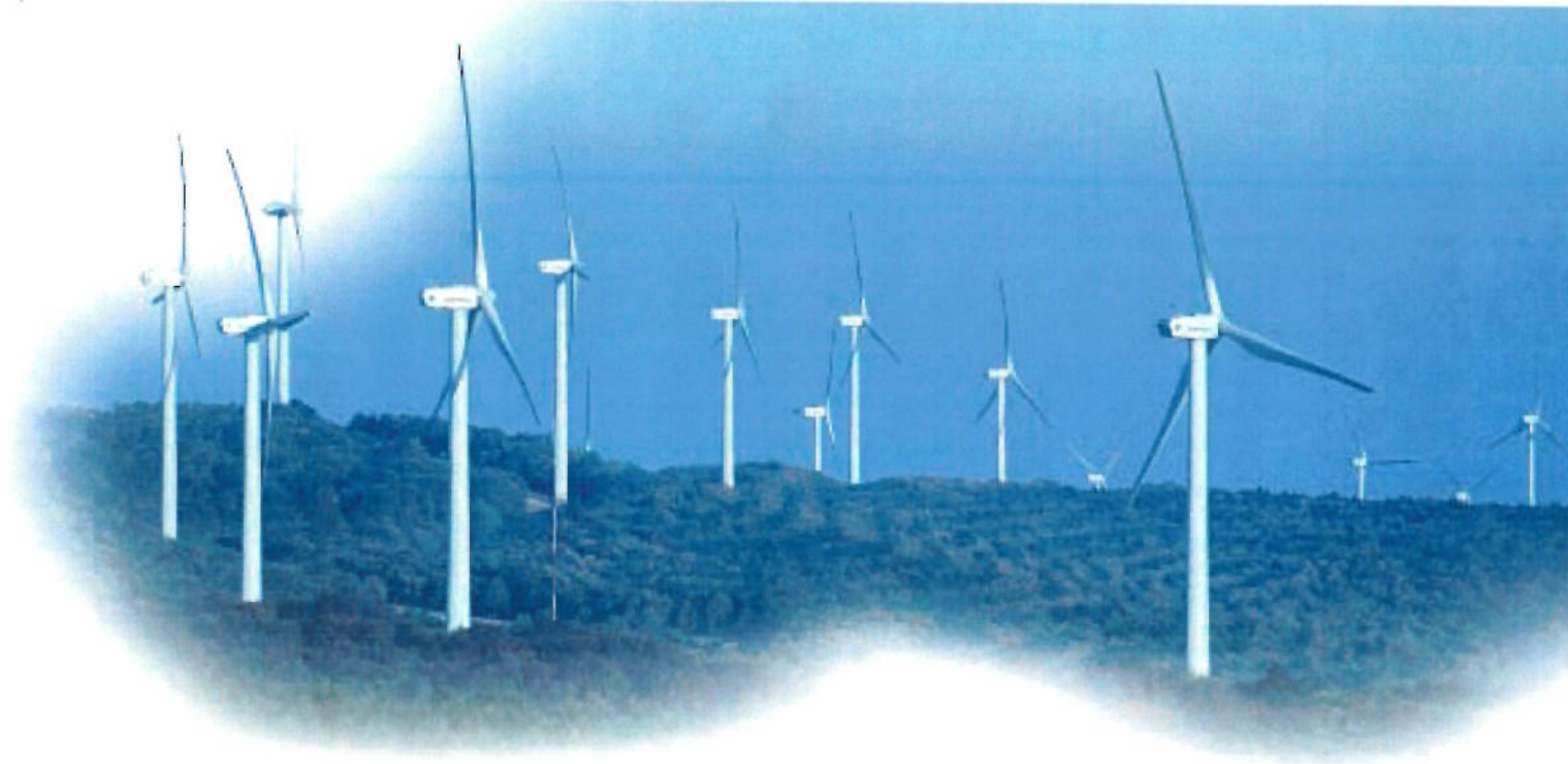
Escorial, Spain 33 x 1.5M total capacity: 49.5 MW
