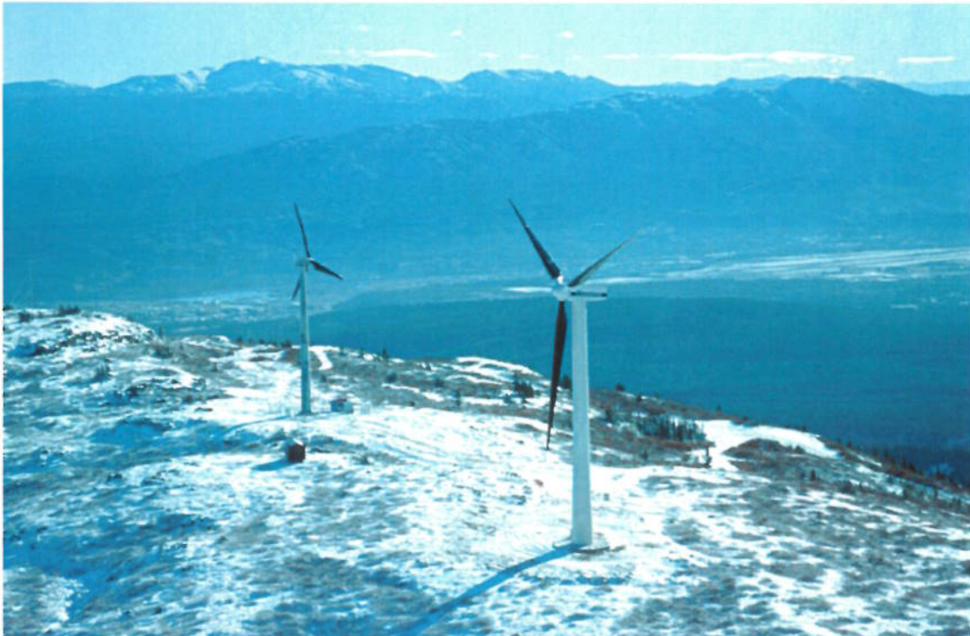
Photograph 10: both wind turbines in place
