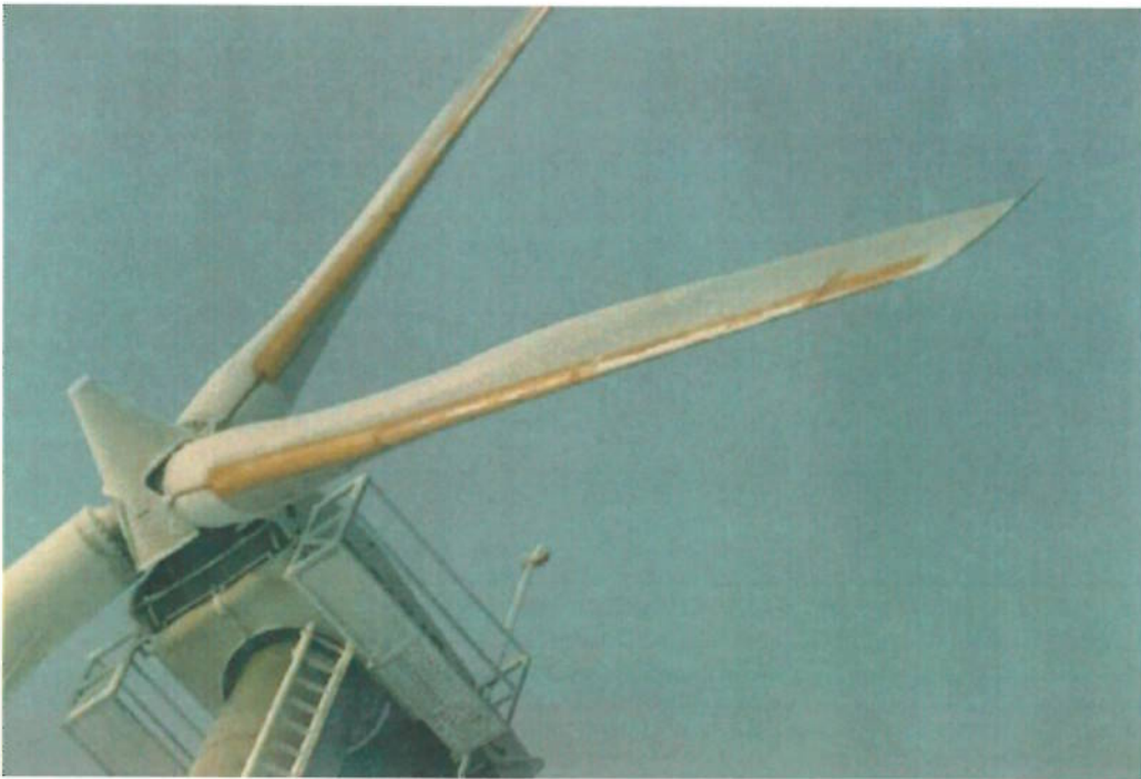
Photograph 6: in less severe rime icing the effect of the leading edge heaters extends past the leading edge
