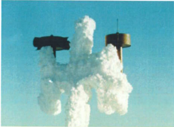
Figure 4. Ice free anemometer in severe icing conditions. (Photo, VTT)
