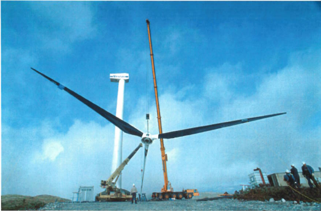
Photograph 9: the second wind turbine being installed
