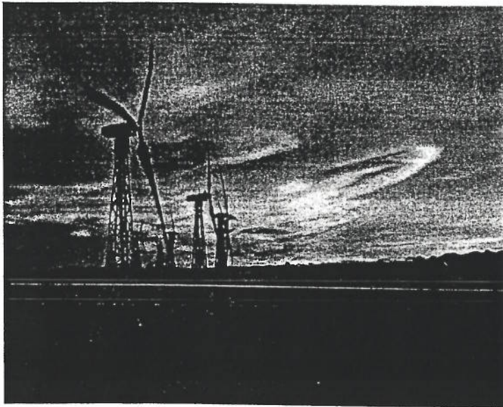
Cowley Ridge Windplant, Pincher Creek Alberta (Photo courtesy of Canadian Hydro Developers, Inc.)
