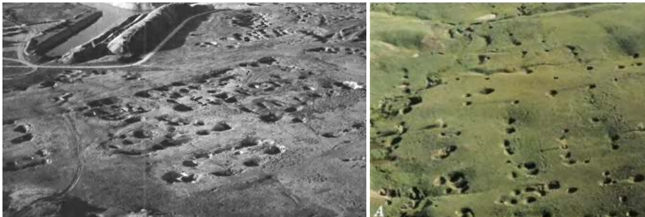
Figure 41. Subsidence and sinkholes at Sheridan, Wyoming from an abandoned underground coal mine 40 The Figure was reproduced from Effects of Coal Mine Subsidence in the Sheridan, Wyoming, Area By C. Richard Dunrud and Frank W. Osterwald Geological Survey Professional Paper 1164, 1980
