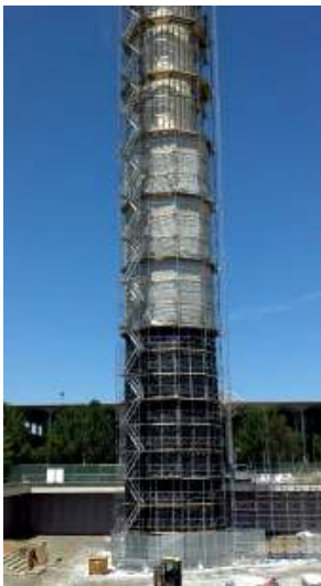
Figure 45. Noise Enclosure for a drill rig 76 Figure was reproduced from reference 76.
