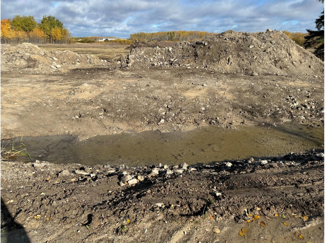
“In water” works at South Malonton Drain Road 106 N(photo taken October 13, 2025)
