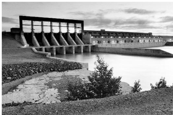
The Limestone Generating Station on the Nelson River. Renewable energy sources supply close to 25 per cent of energy consumed in Manitoba. Photo courtesy Manitoba Hydro.
